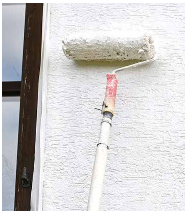
Rehabilitation with GM6-L on Crepi
