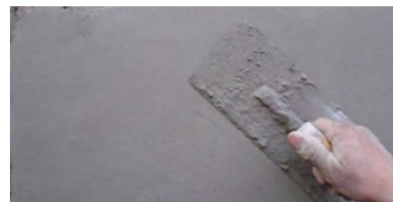
Wall preparation with MAGH
