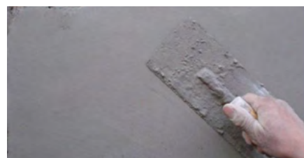
Wall preparation with MAGH
