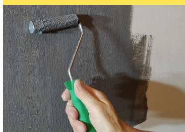
Cementitious mortar application
